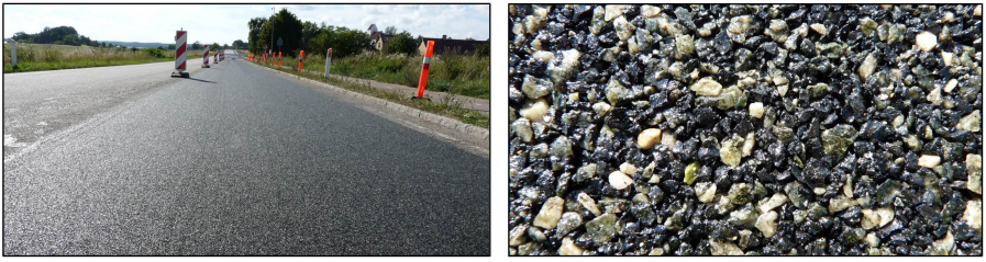
Figure 9: The Kalvehave I full scale test track (August 2013)
