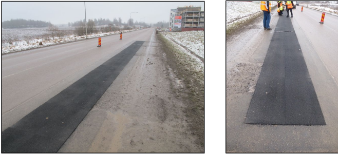
Figure 12: Swedish full scale test track constructed with PERS prefabricated slabs in Linköping in February 2014 (PERS slabs only applied in the right hand wheel track)
