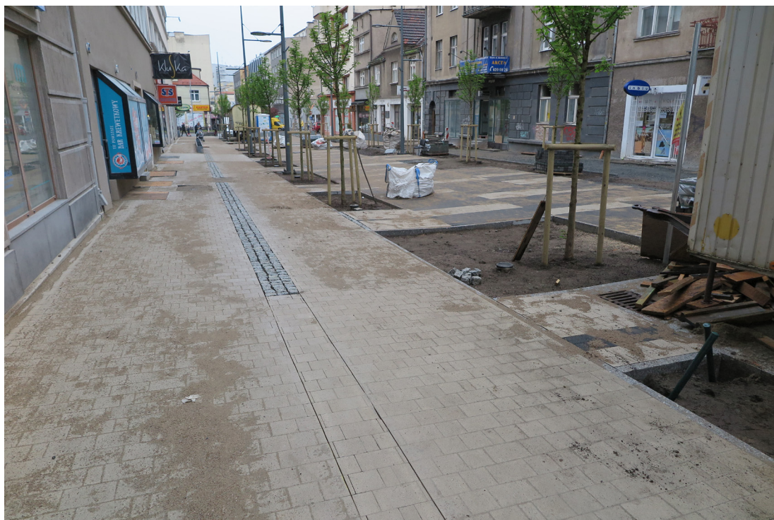
Fig. 5. Gdynia, Abraham Street, the section between Batorego Street and 10 Lutego Street, during the redevelopment into a so-called woonerf; photo from the archives of the Municipal Conservator's Office.
