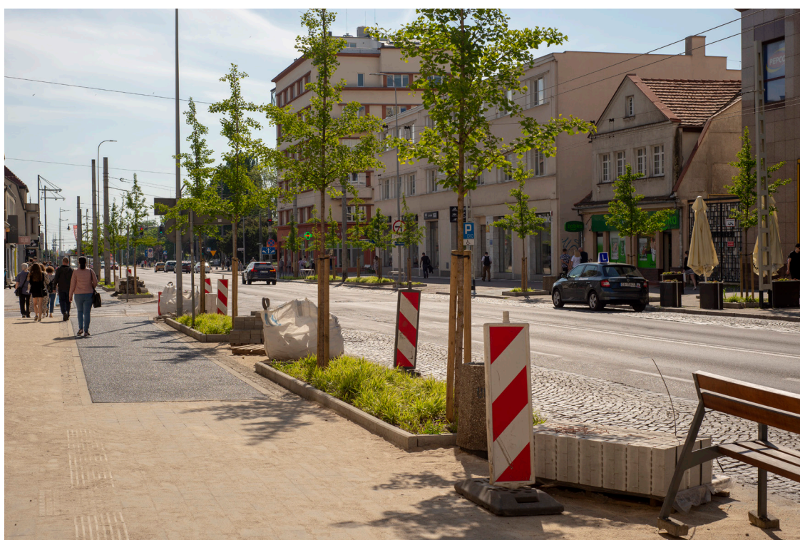
Fig. 3. Gdynia, 10 Lutego Street, after renovation works, which included the conversion of parking bays as well as the reintroduction of the historic width of pavements and the replanting of trees; photo by B. Ponikiewski.
