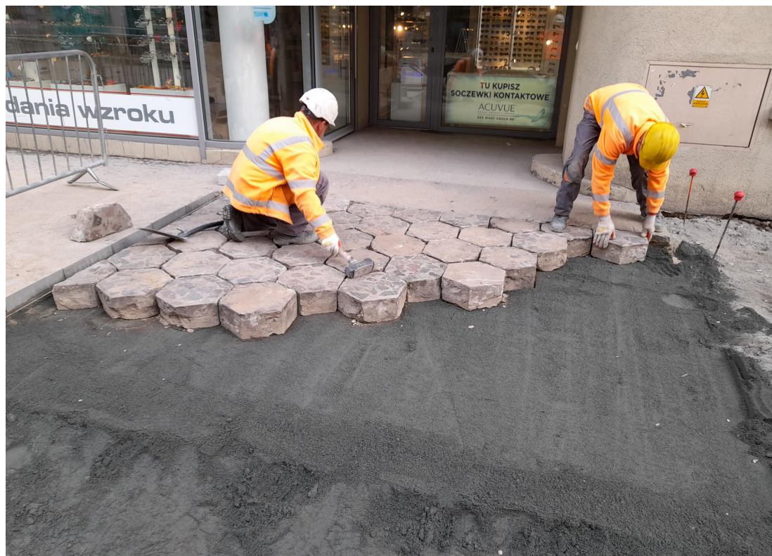
Fig. 4. Gdynia, Starowiejska Street during renovation works in 2022, which involved relocating the historic surface made of hexagonal blocks; photo by R. Hirsch.
