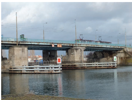
Fig. 1. Siennicki Bridge in Gdansk
