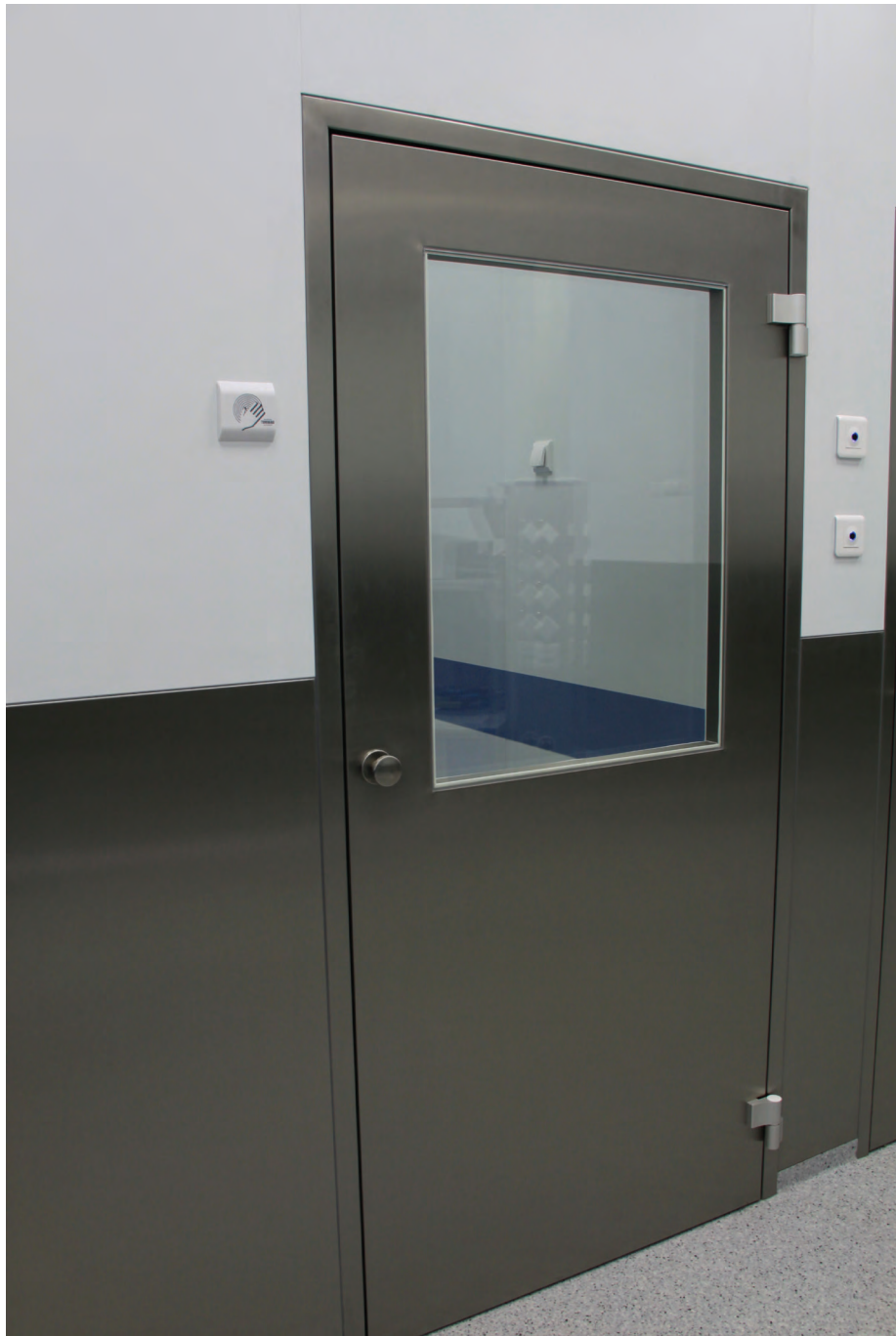
Photograph 6.2.2 Automatically opening door (a solution that reduces a possibility of contaminating medical personnel's hands); photographed by the Author, 2015
