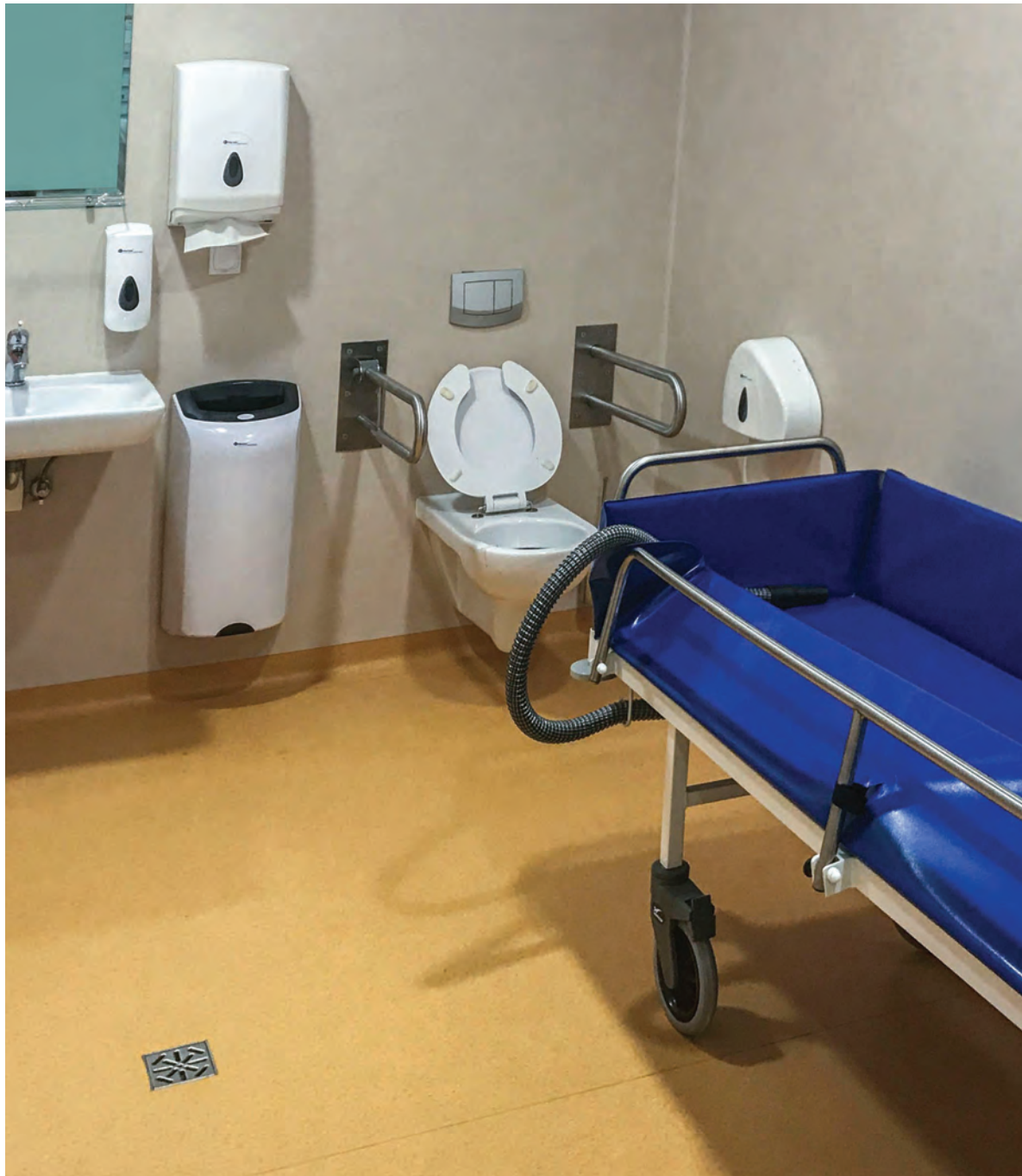
Photograph 2.0.1 A bath trolley – a station for washing patients (a solution that allows for hygienic procedures, e.g.: decontamination of patients during their admission to the area of the hospital emergency department); photographed by the Author, 2016
