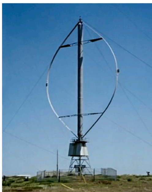
Fig. 1. Darrieus turbine (photo: Aarchiba).
