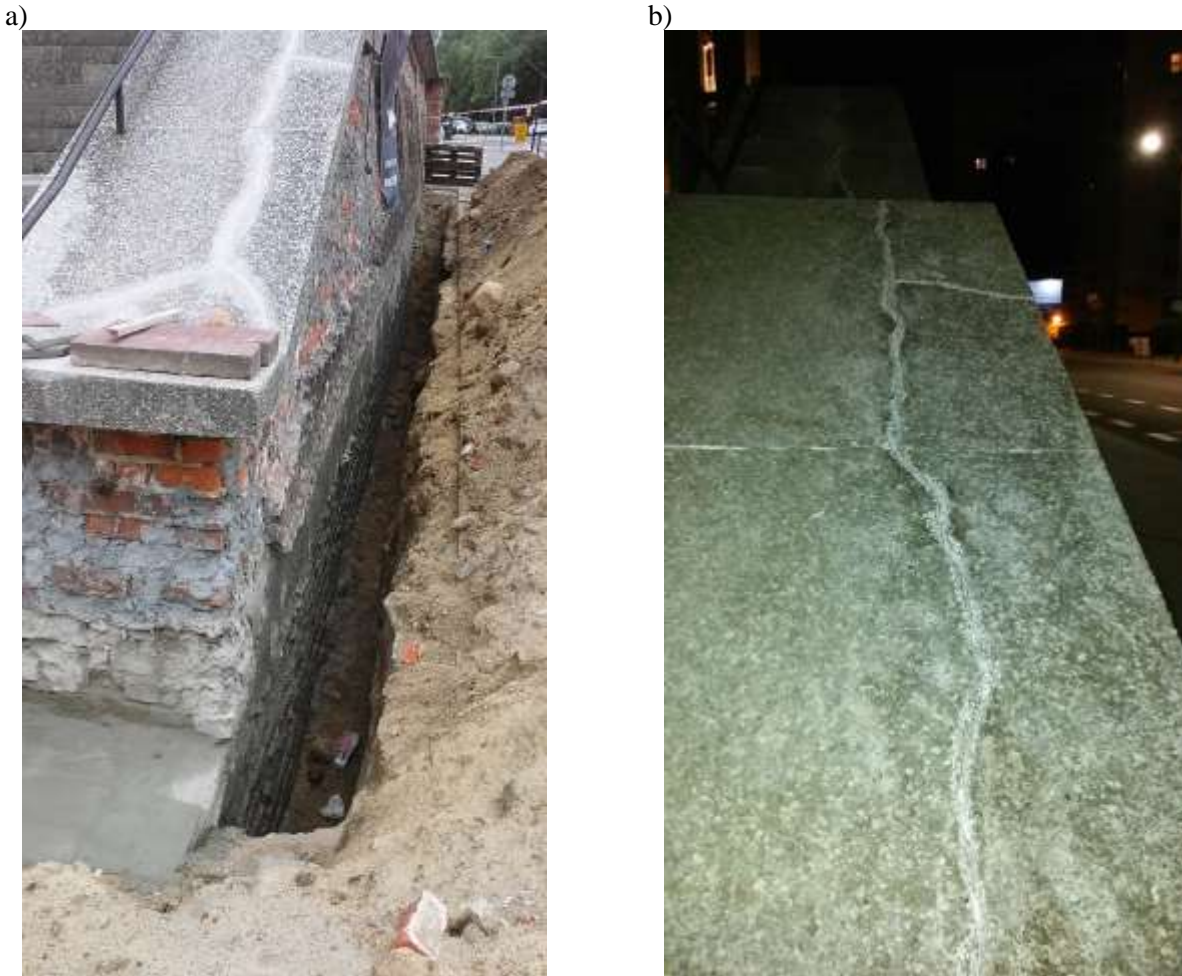
Photo 14. The wall at the entrance from the west elevation (along 3 Maja Street) during renovation works: a) dismantled cracked stone cladding and implementation of vertical damp-proof insulation, b) repaired cracks in the terrazzo cladding of the wall cap (names of the street as of 2023) (photo by Jacek Bramorski)
