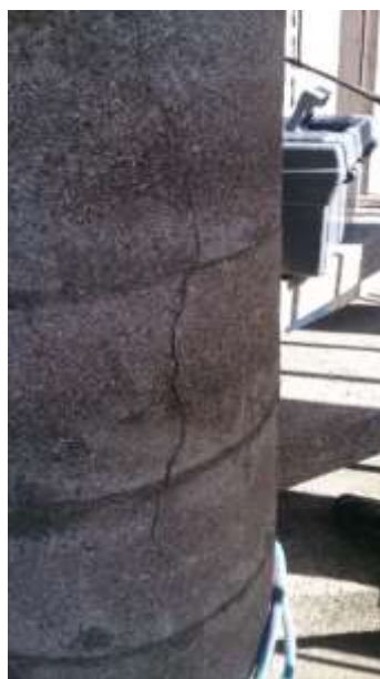
Photo 5. Outlined, in the line of the axial anchorage, prefabricated steps of the spiral stairs leading to the top of the belfry tower (photo by Maciej Niedostatkiewicz)
