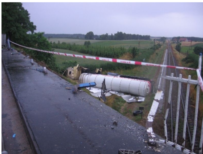
Fig. 1. Fall from the viaduct of the car - a cistern with 20t of propane-butane gas (source: Provincial Police Headquarters - Gdańsk).
