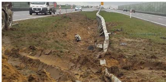
Figure 5. Examples of crashes into road restraint systems (source: GDDKiA)
