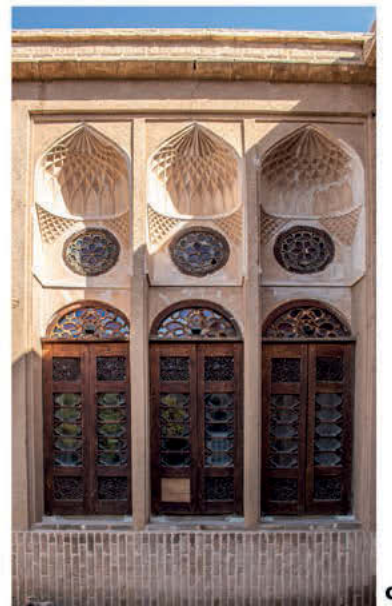
III. 4. Daylight Controllers: a) ravaq in the old fabric of Shiraz (30 October 2021, 4:00 p.m., geographical location: 29.6136, 52.5378, clear sky). b) Sabat in the old context of Yazd (25 October 2021, 12:00 p.m., geographical location: 31.9014, 54.3677). c) External shading system including a tabeshband (vertical fin), a sarsayeh (horizontal fin), and a kharakpoush (arched fin) in the Ameriha House in Kashan (22 October, 2:00 p.m., geographical location: 33.9754, 51.4416, clear sky). A hurno as a skylight in the Aminoddoleh Caravanserai in Kashan. (20 October 2021, 9:00 a.m, geographical location: 33.9843, 51.4488, clear sky type). Source: photos by Mosleh Ahmadi).
