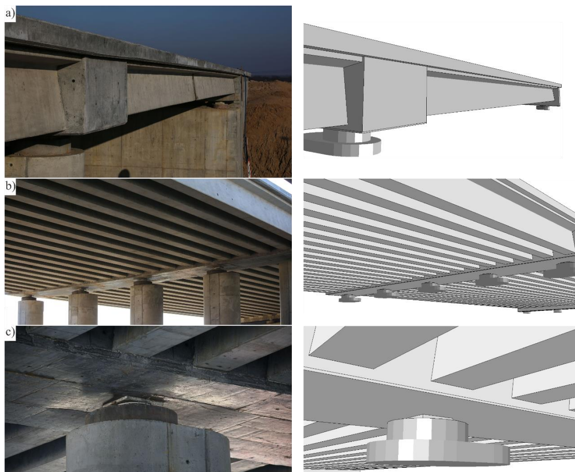
Fig. 8 Comparative views of the viaduct, a) side view, b) bottom view, c) detail of the structural support.
