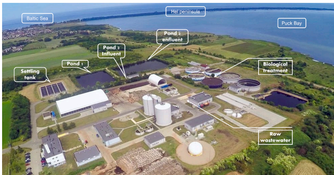
Fig. 1. Scheme of WWTP in Swarzewo with biological treatment tank (SBR), settling tank, pond 1 and 2 with its influent (raw wastewater) and effluent points.
