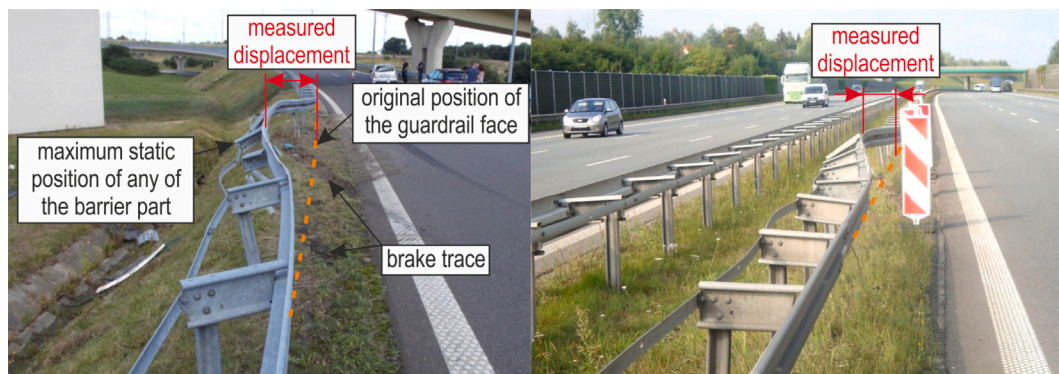
Fig. 5. Examples of measurement of the displacement from the crash scene, source of photos: GDDKiA, Poland.
