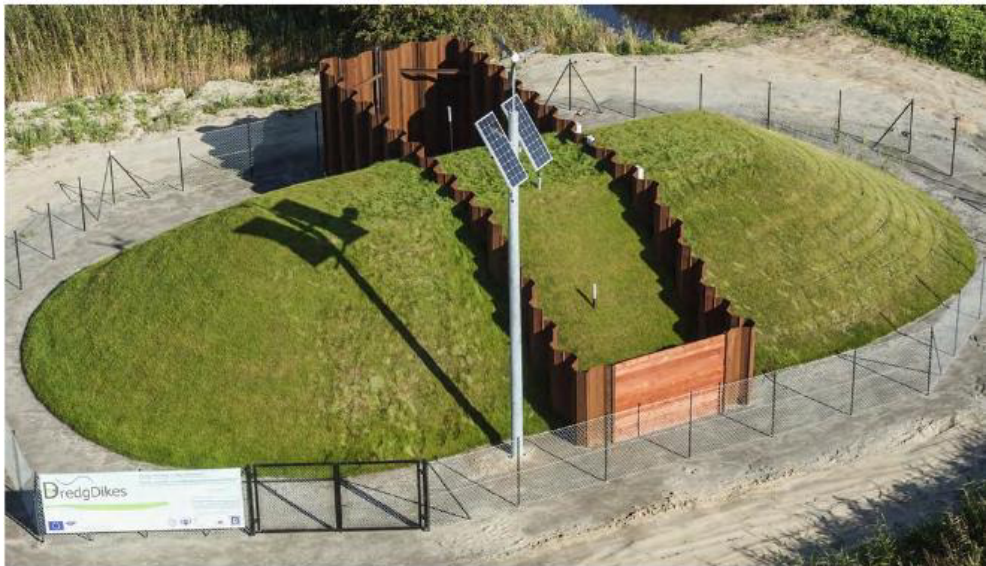
Fig. 1. Test dike in Trzcińsko - near Gdańsk [8].
