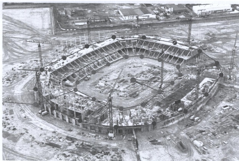
Fig. 11. Vertical geodetic network on the construction site of the stadium.
