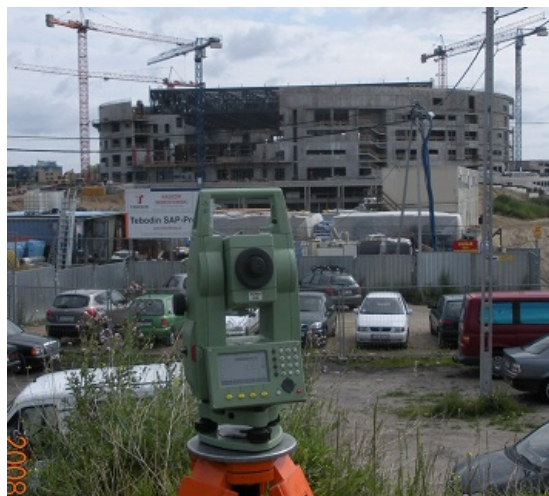
Fig. 2. View of Hall ERGO-ARENA under construction on the administrative border of Gdańsk and Sopot.
