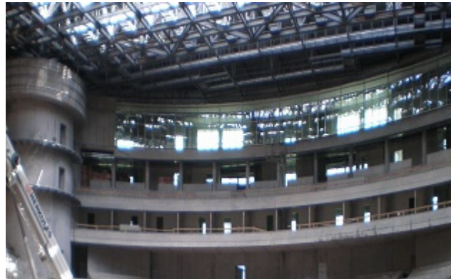
Fig. 3. View of the pylon and the girder of Hall.
