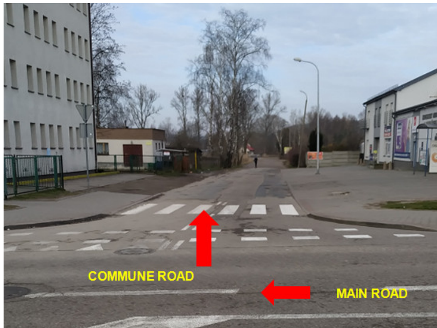
Figure 3. The current solution of connecting the main road with the commune road.
