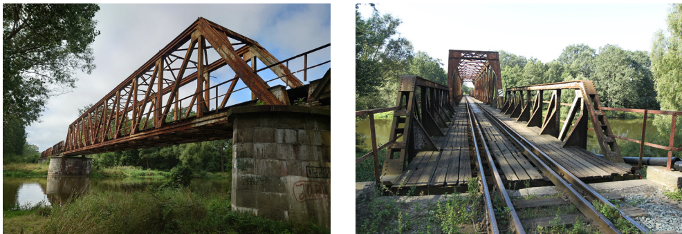
Figure 1. View on railway truss bridge
