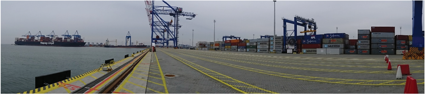
Fig. 12. State of the monitored quay in November 2016
