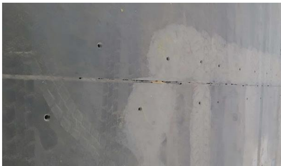
Fig.15. Concrete industrial floor (Example 4) during repair: diagram of drilled holes for injection feeding [38]
