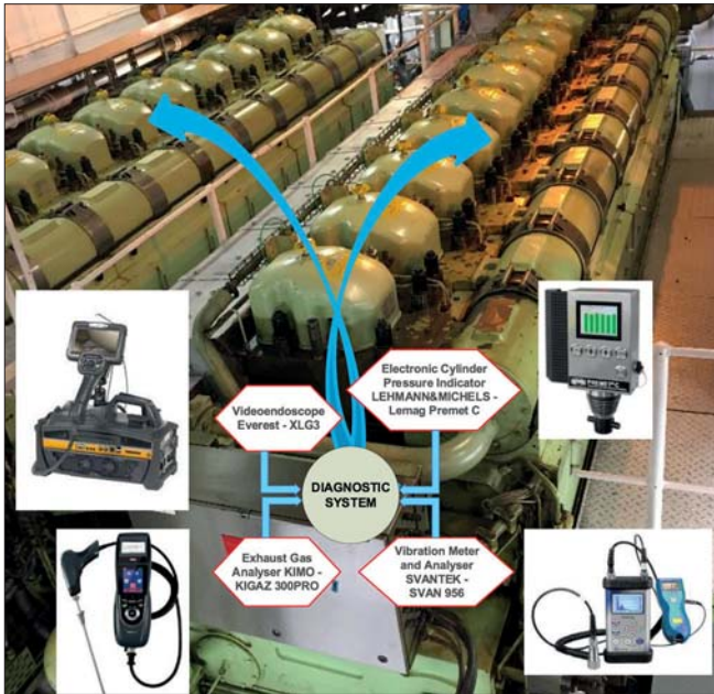
Fig. 1. General view of MAN Diesel 10L32/44CR engines installed in a marine power plant, along with a portable diagnostic system applied to exhaust emission operational tests
