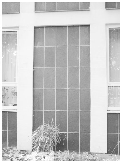
Photo 11. Detail of the clinker façade of Employment Office (Kieler Str.)
