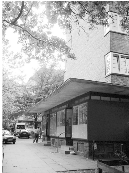
Photo 4. Housing complex Bunsenstrasse
