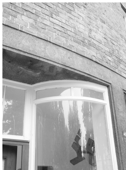
Photo 7. Multifamily building “Schichttorte” – detail
