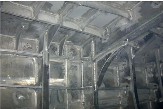
Fig. 1. Typical T-joints in ship structure
