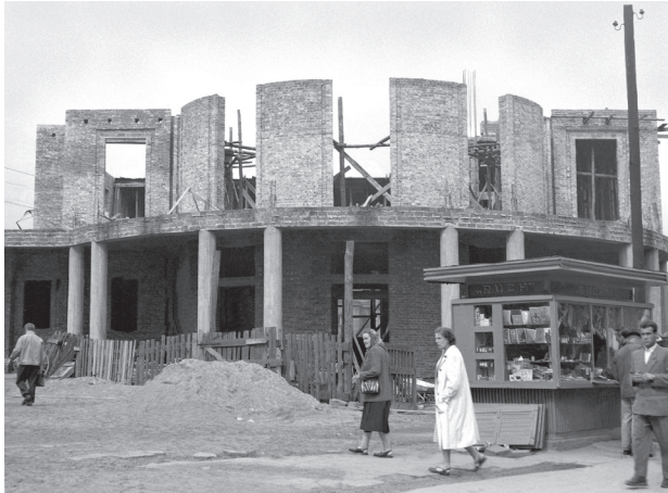
Fig. 2. The new building of the electric railway station in Gdynia under construction, 1958 (KFP) (photo by Z. Kosycarz)
