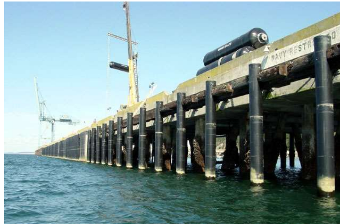
Fig. 2. CFFT piles protecting the wharf from ships mooring at the Hadlock military port on Indian Island, Washington, USA [6], [9]
