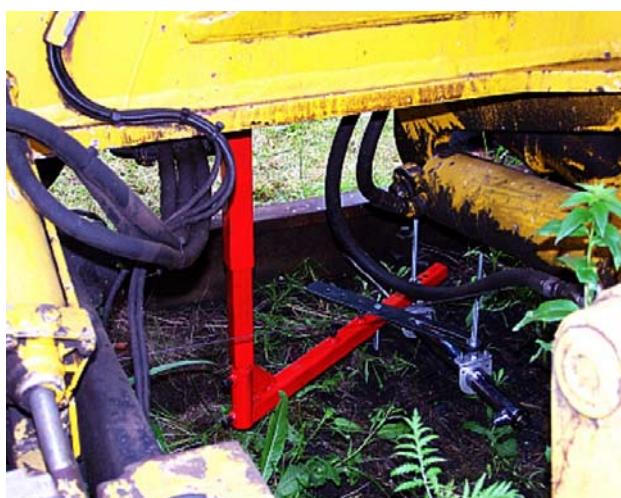
Fig. 13 CL70-200 inductive sensor mounted by the support frame close to the slewing position.
