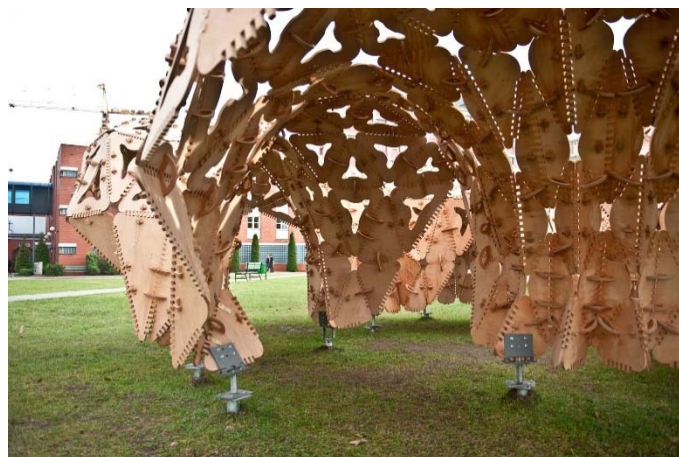
Figure 6. Pavillon was made of plywood panels [38]
