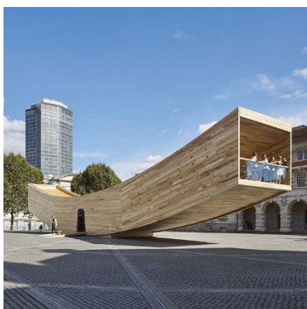
Figure 3. Curve shape was connected with a ground in a narrow, central section [35]
