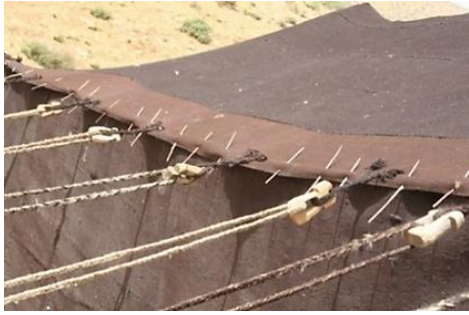
Fig. 85: Wall and roof of the tent are connected by wooden pins, photo by author
