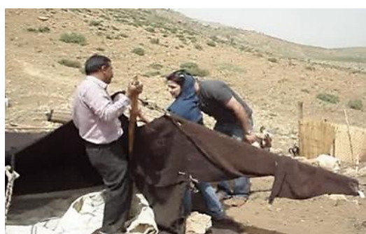
Fig. 77: Qashqai Tribe in Fars Province. Pitching the roof by lifting the end columns, photo by author
