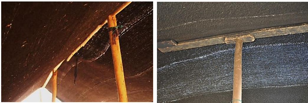
Fig. 93: Qashqai Tribe, Fars Province, two kinds of ridge support by a column, photo by author
