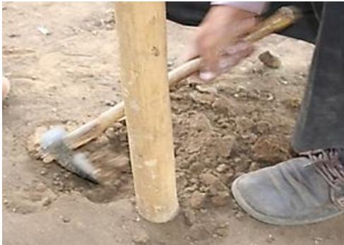
Fig. 82: Digging the end column into the ground, photo by author
