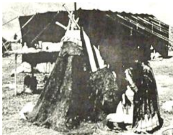
Fig.50:View of bathroom, source: Kiani, M., 1997, p. 88.
