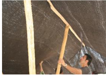
Fig. 80: Lifting the middle column with the ridge beam, photo by author
