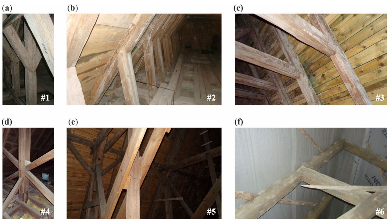
Fig. 6 Carpentry joints in church roof trusses: a Mitobądz (#1), b Pruszcz Gdański I (#2), c Kiezmark (#3), d Pruszcz Gdański II (#4), e Koźliny (#5), f Trutnowy (#6)
