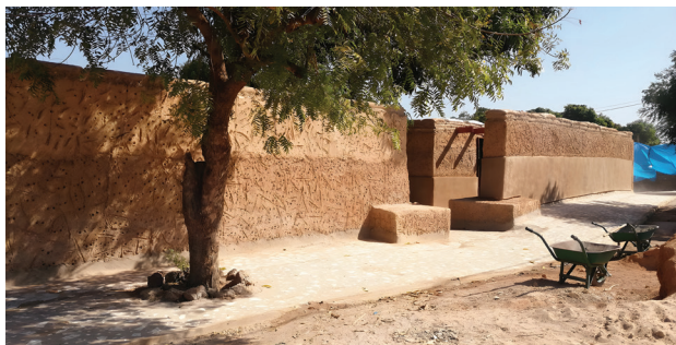
Fig. 1. Polyvalent Cultural Centre, Tanaff, Senegal. In the construction phase
