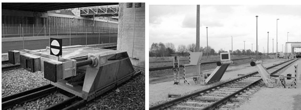
Fig. 4 Buffer stop with impact energy-absorbing buffers [4, 6]
