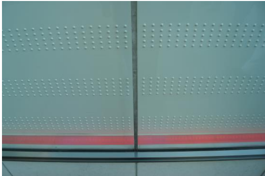
Fig. 15 Matsuya Ginza – detail of the curtain wall
