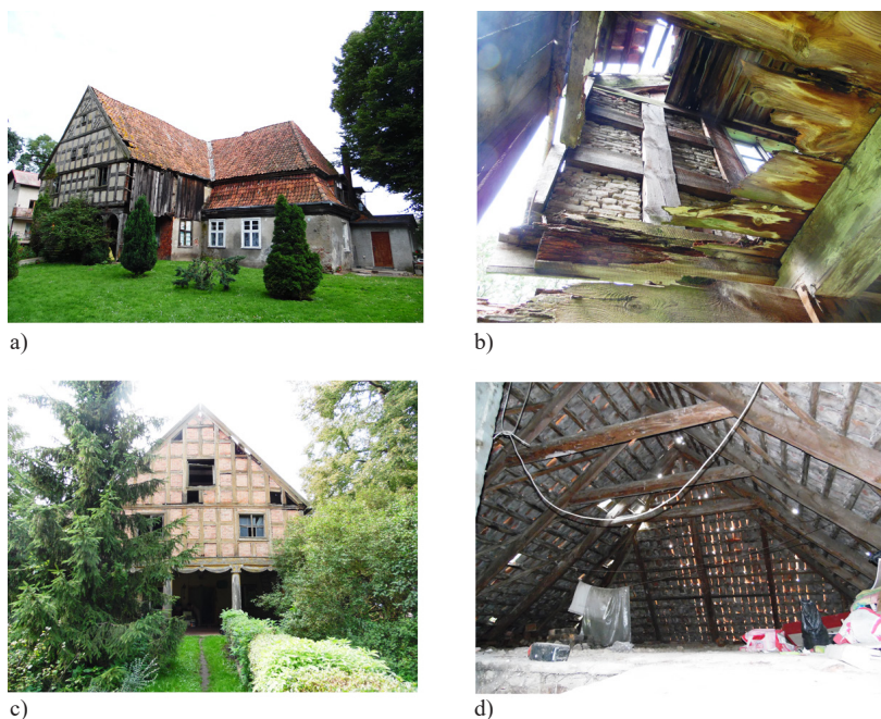
Fig. 6. Houses in: a) Steblewo 22/24, b) Steblewo 22/24 the catastrophic condition of the gable wall of the portico, c) Steblewo 15/17, d) Steblewo 15/17 leaking roofing ( photo by the author )
