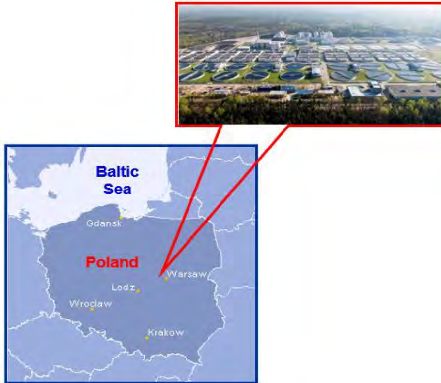
Figure 4- Czapka WWTP in Warsaw, Poland
