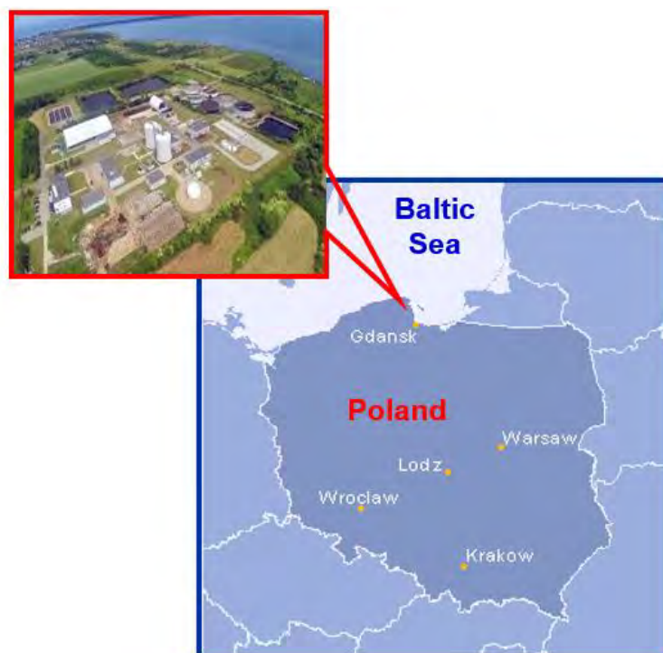
Figure 7- Swarzewo WWTP in Swarzewo, Poland
