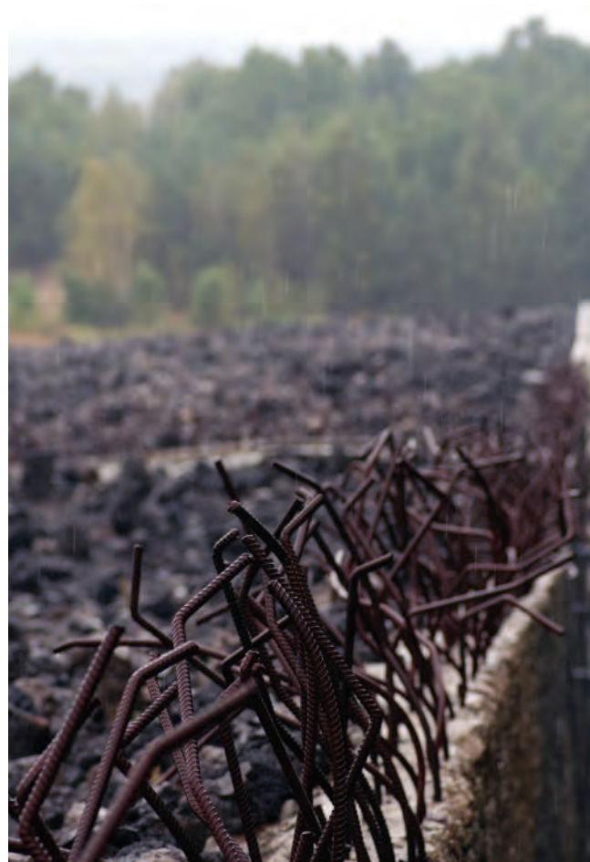
8. Reinforcing bars at the top of the wall
