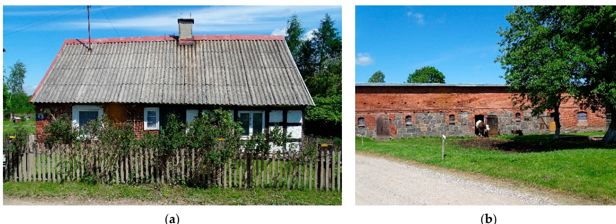
Figure 3. Historic farm buildings in the study area: (a) a house of mixed construction (of brick, half-timbered) with a high, steep roof; (b) a cowshed of brick and stone with a semi-flat roof (photos by A. Górka).
