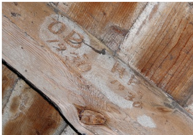
Figure 3. A rafter at the top of the roof of the monastery's west wing. (Hliwiadczyń, Cholewska, and Grunwald 2018).
