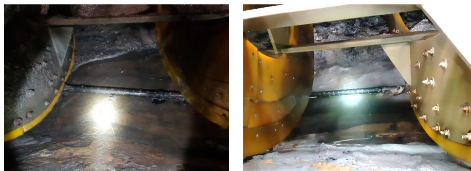
Figure 16. View of selected polarization anodes installed in a perforated ABS cover.
