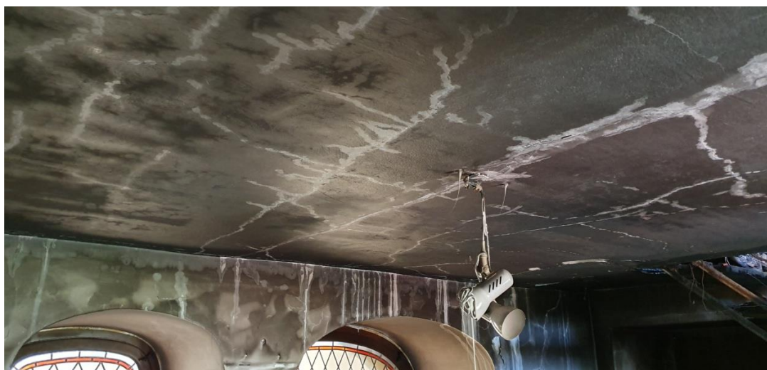
Fig. 5. Fire damage to solid ceramic brick wall and ceiling on wooden beams, visible cracks in plaster on wall and ceiling (photo: Maciej Niedostatkiwicz)
