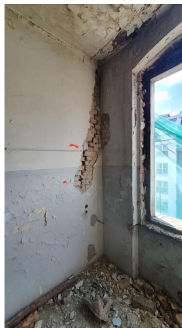
Fig. 11. Cracking of the internal transverse wall made of solid ceramic bricks at the point of connection with the exterior longitudinal wall in a building with ceilings on wooden beams that do not have frontal and lateral anchoring (photo: Maciej Niedostatkiwicz)
