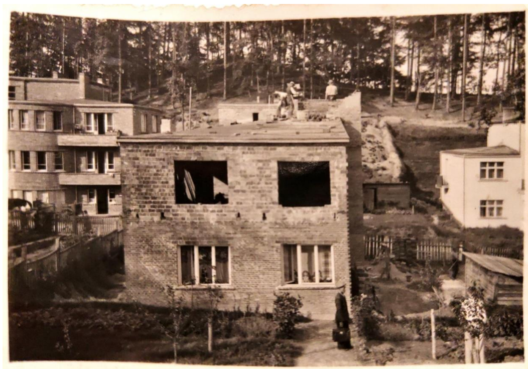
Fig. 12. Building with layered exterior walls (with air cavity), made of ceramic bricks: a) solid, at the level of the ground floor, b) trusses, at the level of the first floor (photo: Jan Niedostatkiwicz)
