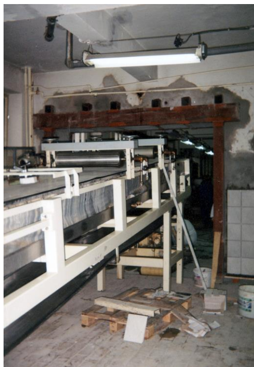
Fig. 18. Widening of the door opening in the inner wall of solid ceramic brick – view of the steel frame construction (photo: Maciej Niedostatkiwicz)
