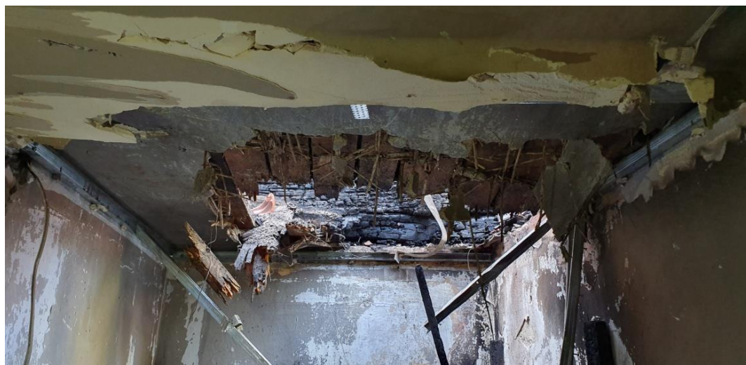
Fig. 14. Moisture damage to exterior and interior ceramic walls as a result of water flooding at the site of a broken roof (photo: Maciej Niedostatkiwicz)
