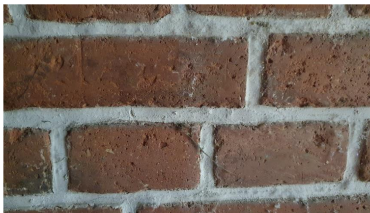
Fig. 1. Open pores and capillaries of the exterior masonry of solid ceramic brick, visible cement mortar tight joint improperly executed in the past period during renovation work (photo: Maciej Niedostatkiwicz)
