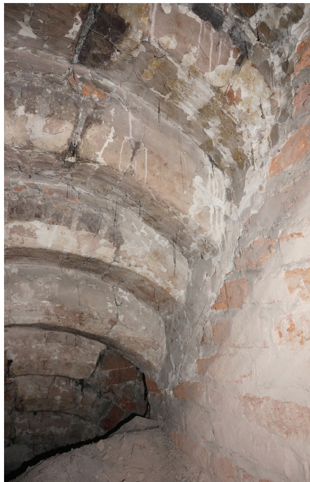
Fig. 5. A section of a partially buried descent from the level of the former matroneum to the ground floor of the chapel at St. Joseph's Church in Gdańsk (photo by A. Piwek)
