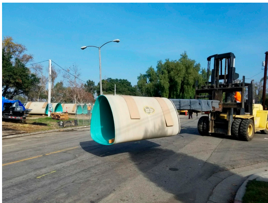
Figure 15. Unloading and transportation of segments of pipe on-site [34].
