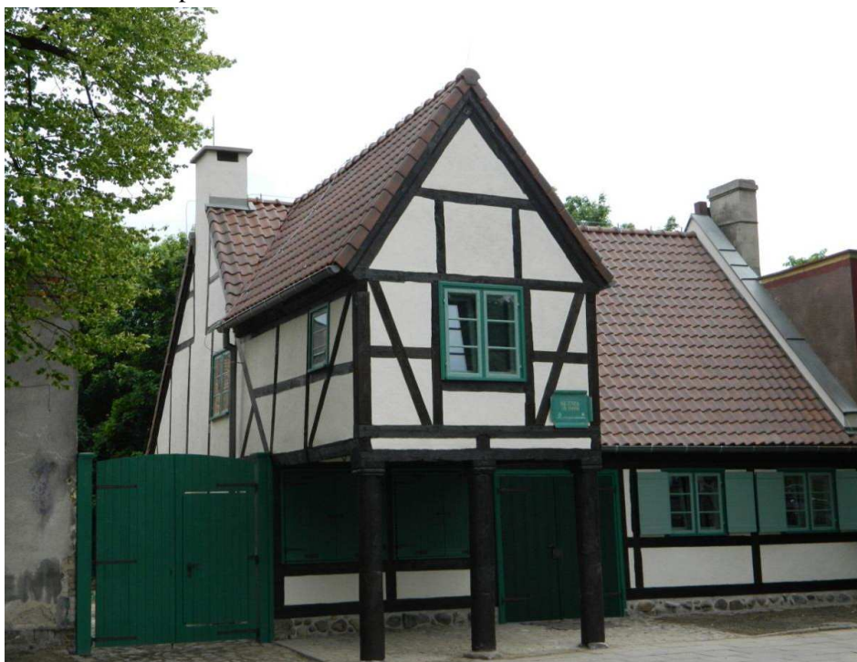
Fig. 1. Forge building after completion of construction-conservation work
