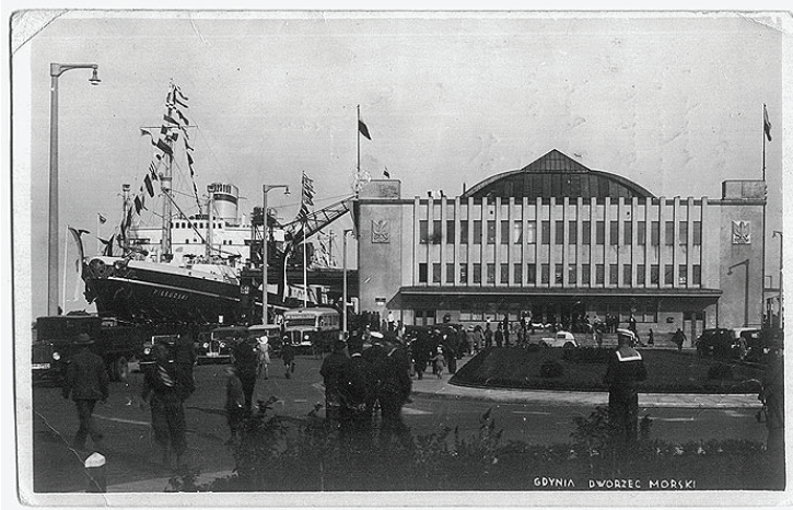
Fig. 1. The Gdynia Seaport Building, 1933 ( http://www.ronet.pl/ )
