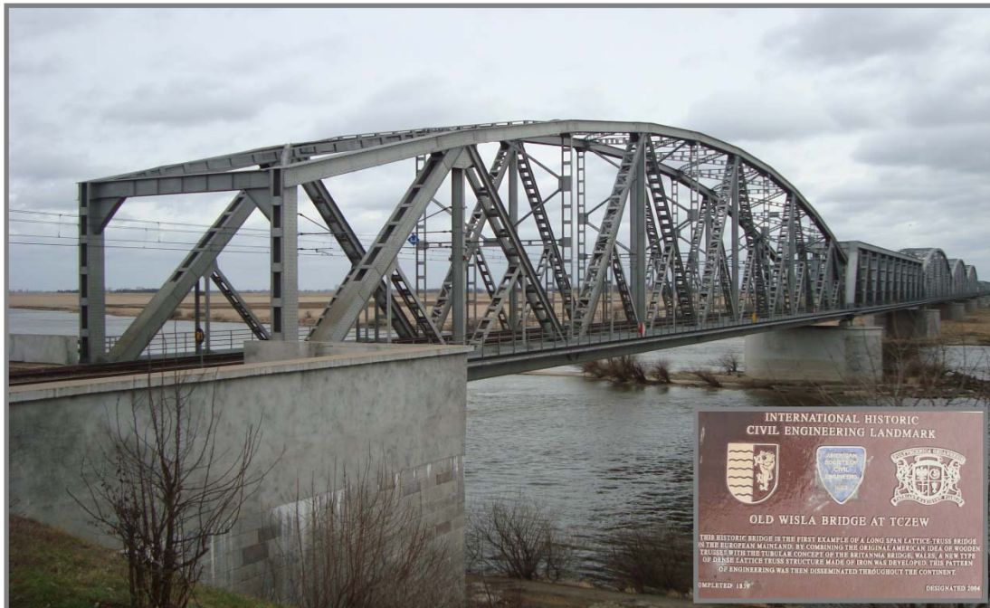
Fig.2. View of the historic railway bridge span no. 10 in Tczew,
