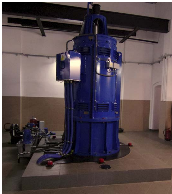
Fig. 2. Tested turbine set in a technical room located in the hydroelectric power plant
