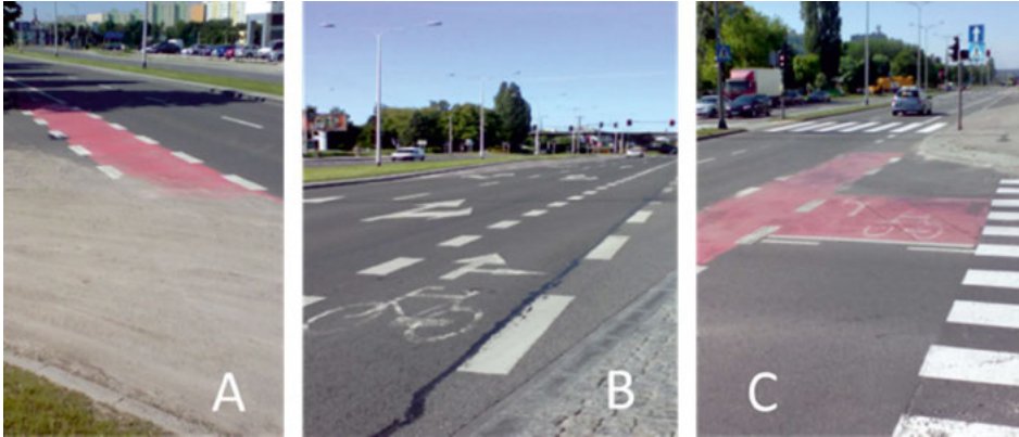
Fig. 4. Cycle lane in Jana Pawła II: a) pools of sand b) horizontal markings far away from one another c) advanced stop line and cycle crossing marked in red
