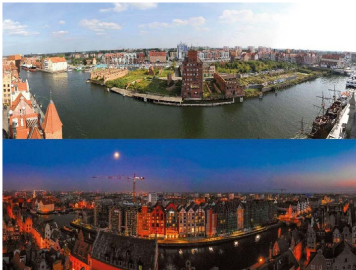
Figure 3. Granary Island – state as of 2012 (top) and of 2019 (bottom)
