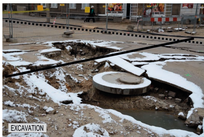
Figure 13. Close-up of the Gdańsk 2013 pipe failure area Dotted lines indicate road edges while solid line indicates the axis of the pipeline
