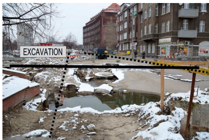
Figure 12. General view of Gdańsk 2013 real-life case of a pipe failure in the vicinity of an unsecured excavation that inspired this study Dotted lines indicate road edges while solid line indicates the axis of the pipeline
