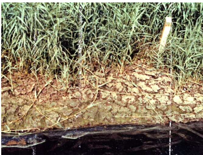
Fig. 1. The sludge drying reed bed
