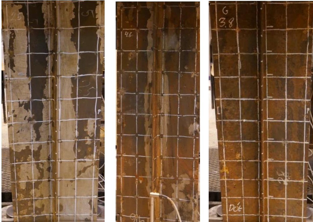
Figure 4.19. Corroded stiffened plates examples - 2.5 (left), 4.6 (mid) and 3.8 (right).
