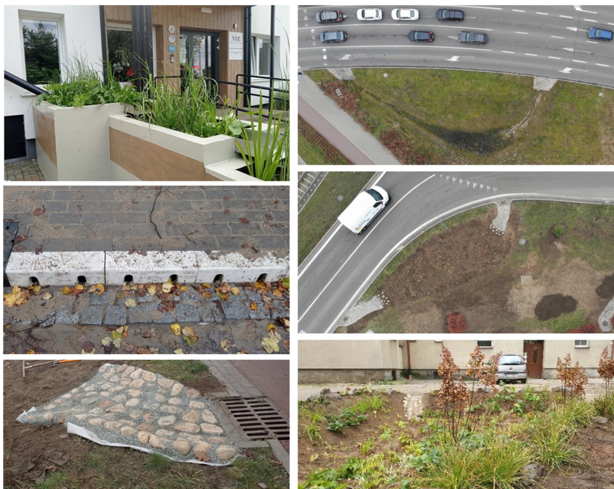
Fig. 4. Examples of simple NBS solutions for stormwater retention from Gdańsk.
