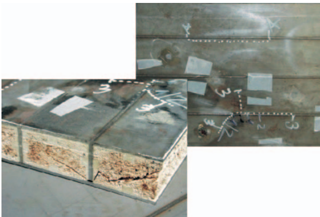
Fig. 3. Fatigue cracks in the model .
